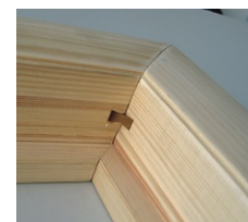
Mitred corner on window frame
