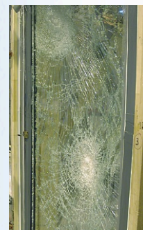
Despite an impact velocity of around 38 mph neither the foil in the laminated glass was pierced nor the corner joints damaged.
